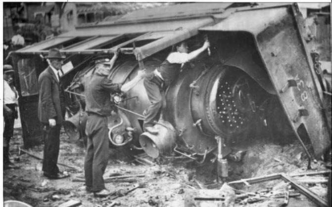
Dismantling motor 83A. The extent of the damage on the lower side readily makes apparent how a driver could be fatally injured.
