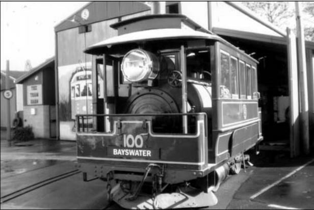
**(Above) Motor 100 looking spic and span outside the depot. Note the absence of a safety-gate in front of the "plough". These were a later innovation made when the motors in NSW were converted to one-man operation.**
