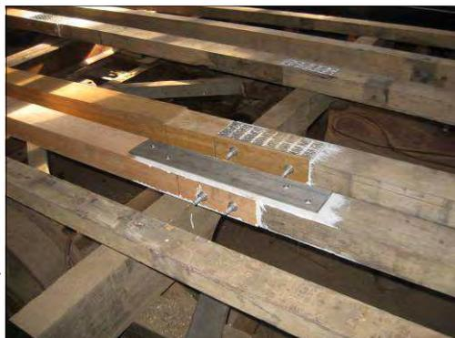
(Above) Detail of splice work done. The splice is additionally supported by hidden knuckle joints and steel plates placed either side.
