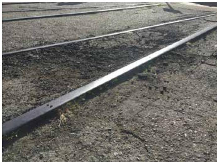
Two views of the current forecourt surface clearly showing the failing uneven surface. The rail head is protruding above the asphalt surface creating a trip and fall hazard. Photos: Andrew Tester
