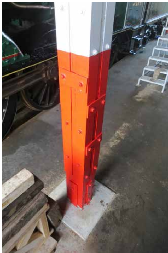
Repaired roof supporting post (Photo: Keith Ward)
