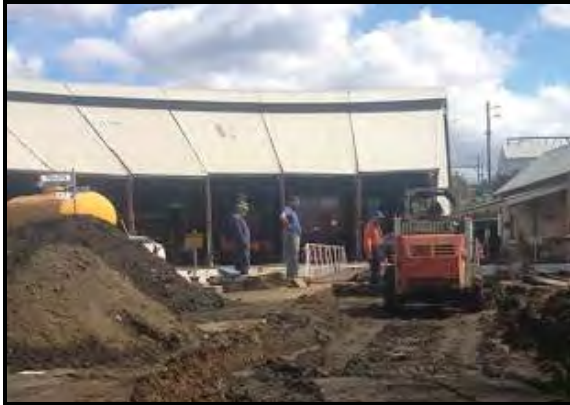
Above: With the Arrival Road lift on the approach to the Turntable, excavation work commences in readiness for the new bed (left) to be laid. Photos: Lee Hawkins.
