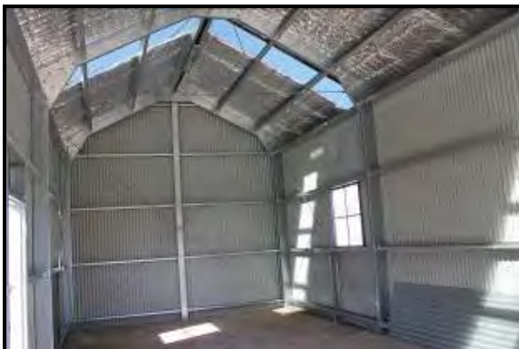
Above: View inside the near completed shed – 5 August 2013. Photo: Andrew Tester.
