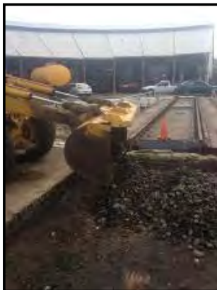
Above: With the Arrival Road lift on the approach to the Turntable, excavation work commences in readiness for the new bed (left) to be laid. Photos: Lee Hawkins.
