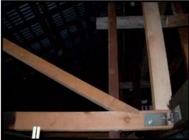
Above: New timber trusses installed by the members of the Retirees Group in the Roundhouse roof above Bay 4. Photo: Andrew Tester.
